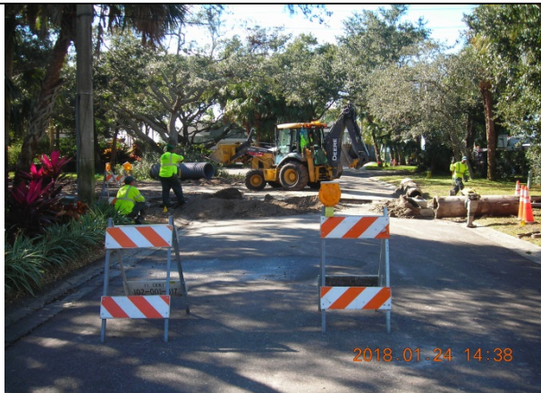
Road Closure at West End of 42 nd Ave for Interconnecting New Storm Drain on Left with Old Drain on Right (next to Canizares Estate)
