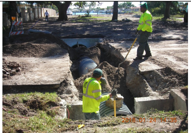
Close-up of Stormwater crew working on interconnection across 42 nd Ave (Main canal can be seen in far background)
